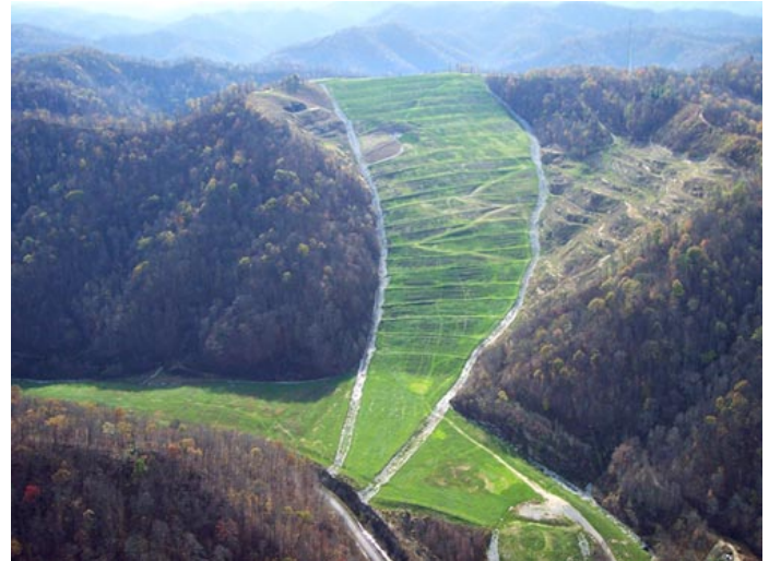
Spewing Camp Project After Reclamation - 2004
