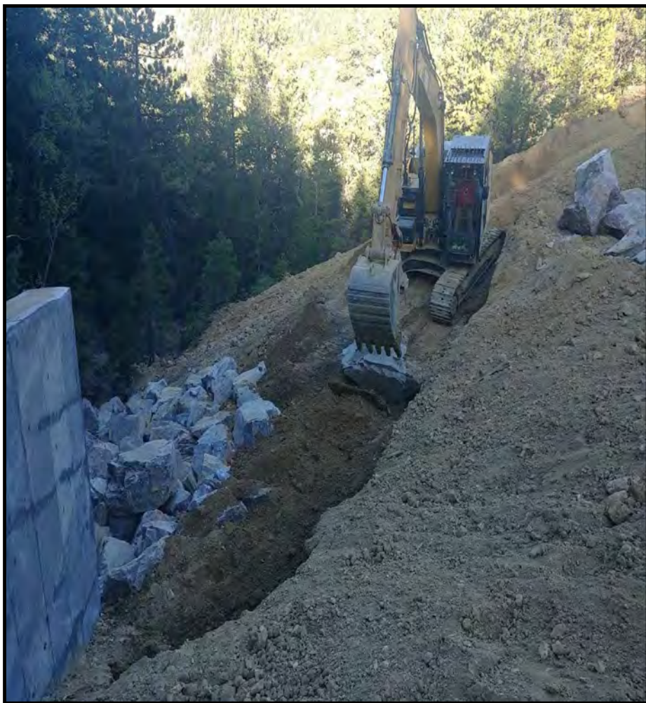
Photos # 23 & 24-Armored Lower Channel Pre and Post-Reclamation
