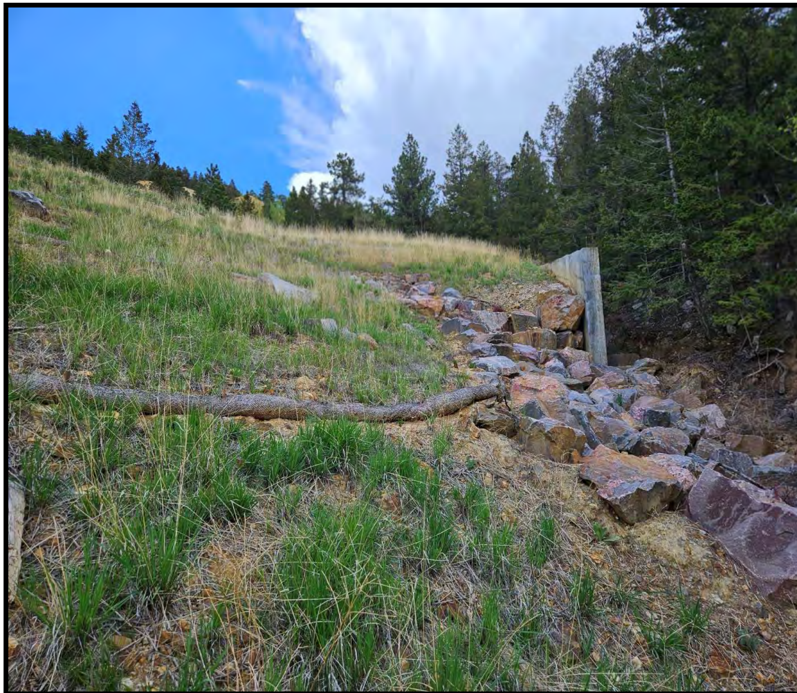
Photos # 23 & 24-Armored Lower Channel Pre and Post-Reclamation
