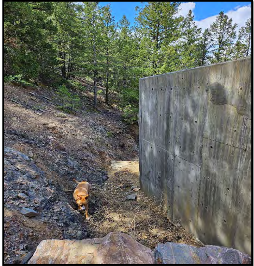
Photo # 7-Upper Concrete Wall Anchored in Bedrock
