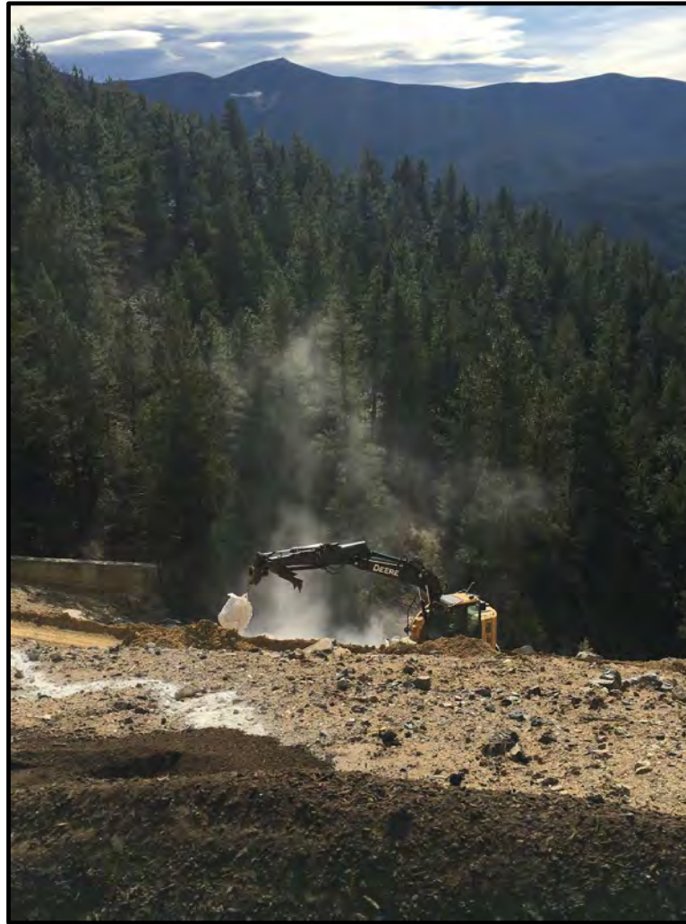
Photos # 29 , # 30 and # 31 - Transporting Crushed Limestone In Supersacs and Spreading Lime with Excavator
