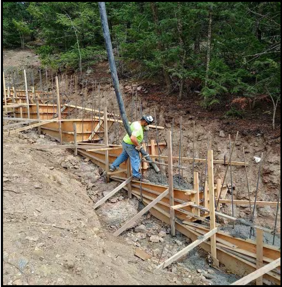
Photo # 4- Pouring Footer-Rebar Dowels Installed
