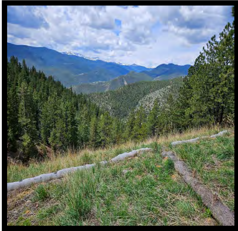
Photo #18 (Left), Final Grade of Waste Pile-. Over 18,,000 cubic yards of material was cut from the top of the waste pile, transported downhill and re-contoured using an excavator and skid steer. It took over 5 months of construction to achieve the final grade. Photo # 19 (Right)- 1.5 Year Post-Reclamation.
