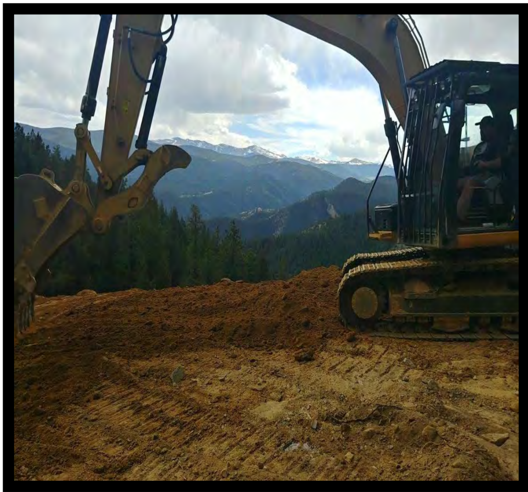
Photo #18 (Left), Final Grade of Waste Pile-. Over 18,,000 cubic yards of material was cut from the top of the waste pile, transported downhill and re-contoured using an excavator and skid steer. It took over 5 months of construction to achieve the final grade. Photo # 19 (Right)- 1.5 Year Post-Reclamation.
