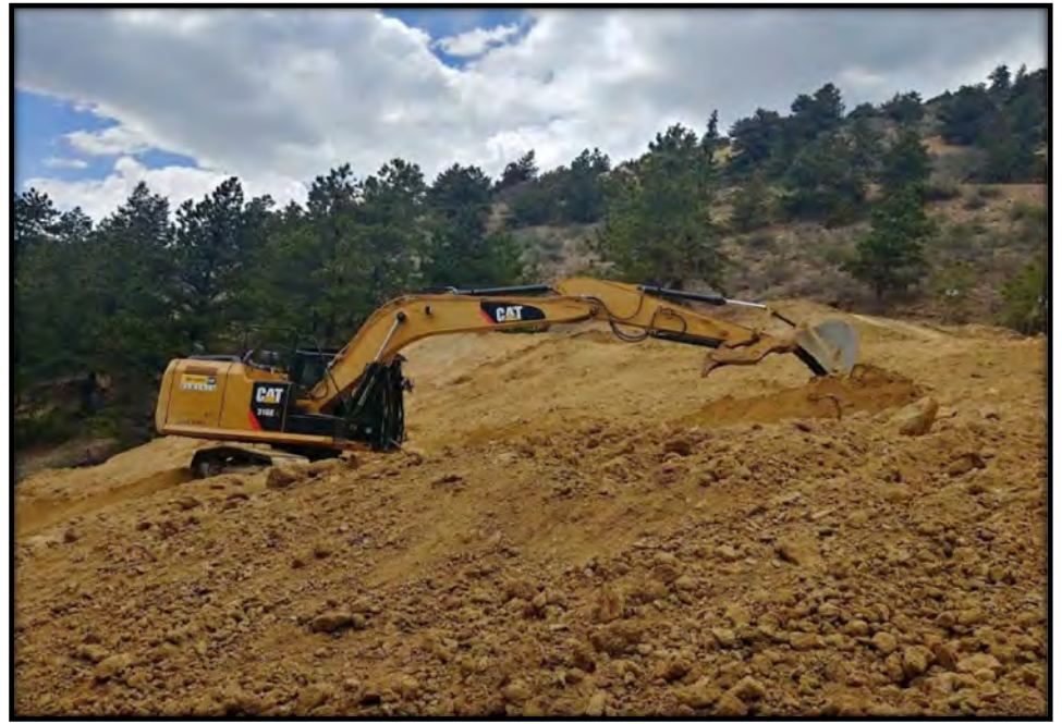
Photos # 14 and 15 -Transporting Material Downhill and Grading Waste Pile with Excavator. Grade was too steep for trucks and dozers. It took over 5 months to achieve the final grade using only a skid steer and excavator to transport and consolidate material.
