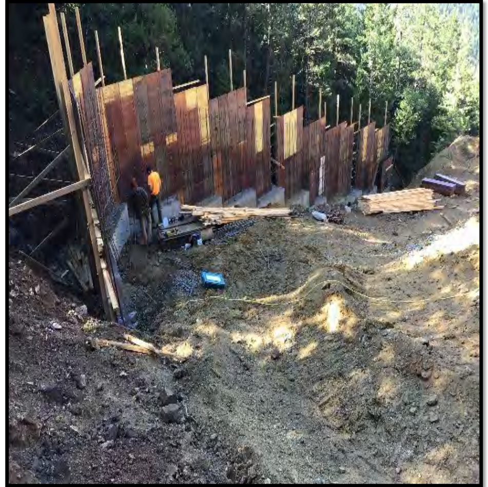
Photo # 5- Forming Wall
