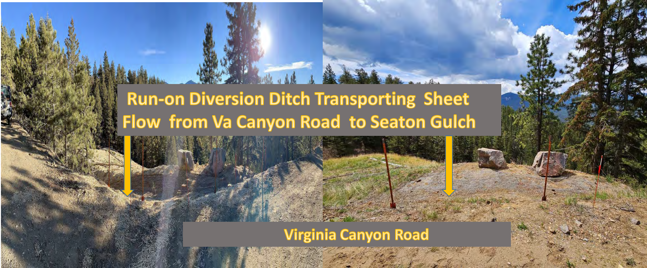
Photos # 39 & 40- Run on Diversion Ditch Pre and Post-Reclamation
