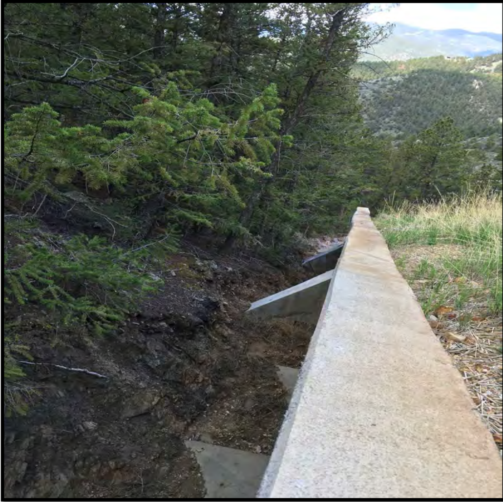
Photo # 6- Counterforts on Concrete Wall
