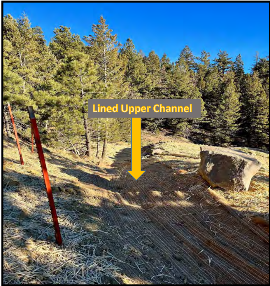
Photos # 37 & 38 -Upper Channel and Run-On Ditch to Divert Sheet Flow from Virginia Canyon Road Around Waste Pile into Lined Channel
