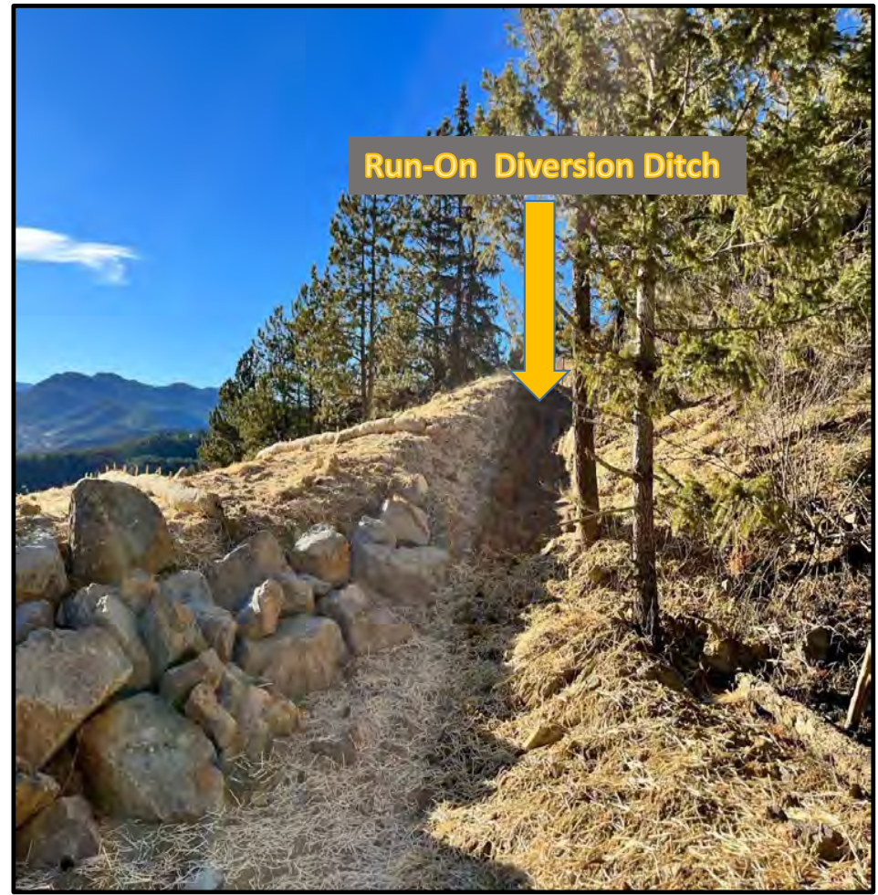
Photos # 37 & 38 -Upper Channel and Run-On Ditch to Divert Sheet Flow from Virginia Canyon Road Around Waste Pile into Lined Channel
