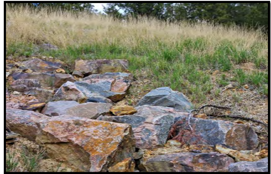
(Lower Right) Photo # 22-Armored Ditch 1.5 Years Post- Reclamation
