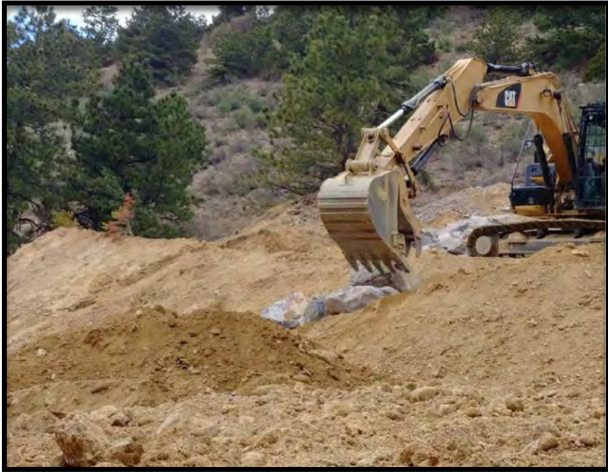
Photos # 14 and 15 -Transporting Material Downhill and Grading Waste Pile with Excavator. Grade was too steep for trucks and dozers. It took over 5 months to achieve the final grade using only a skid steer and excavator to transport and consolidate material.
