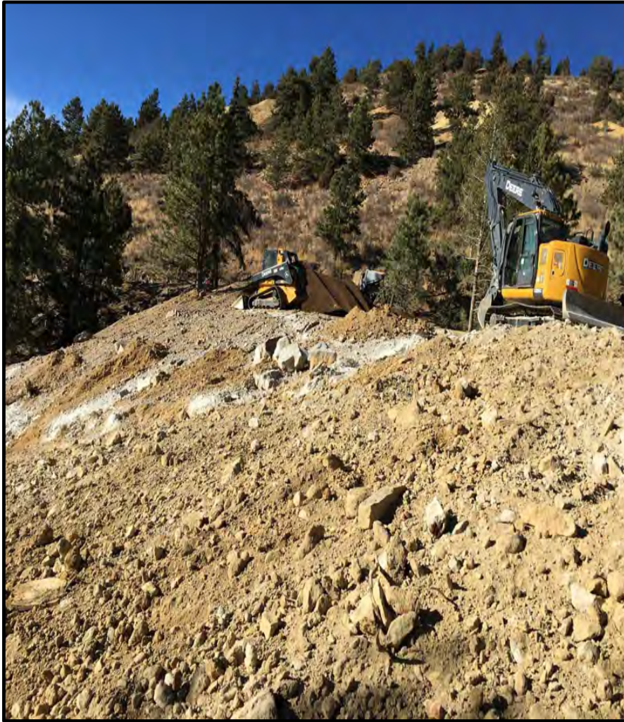
Photos # 33 & 34-Incorporating Lime and Compost with Skid Steer and Hand Labor & Slope 1.5 Years Post Reclamation
