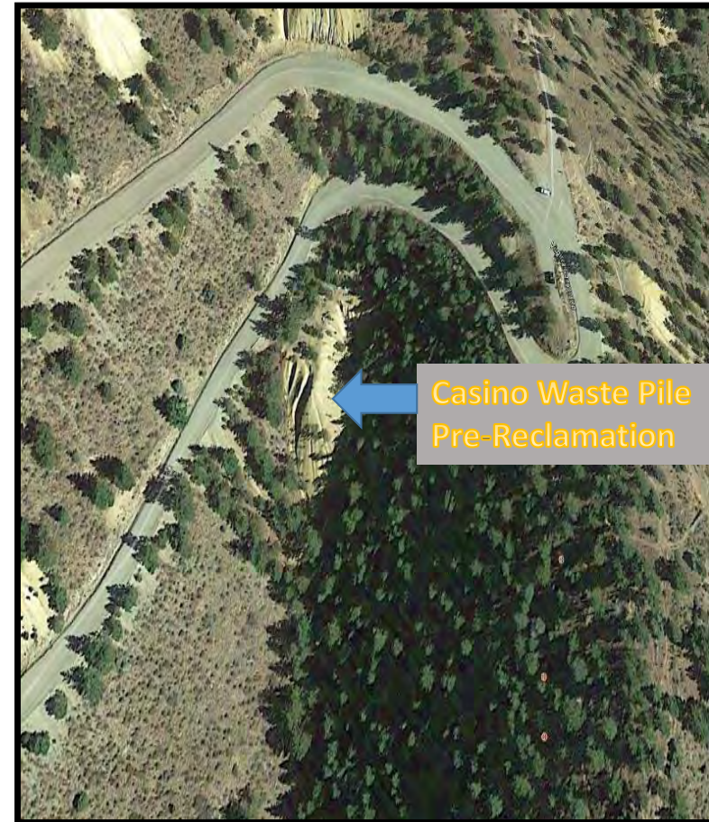
Figure #2- Casino Mine Pre-Reclamation\Access by Steep Unpaved Mountain Road. Steep incised gullies.
