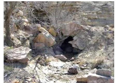
Unreclaimed adit at the Laguna Circle site.
