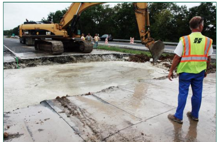
330 cubic yards of flowable fill placed to elevation of pavement subgrade
