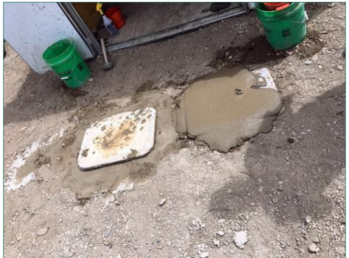
The testing area is on-site, away from the activity. A shed is used to hold the samples for field curing.
