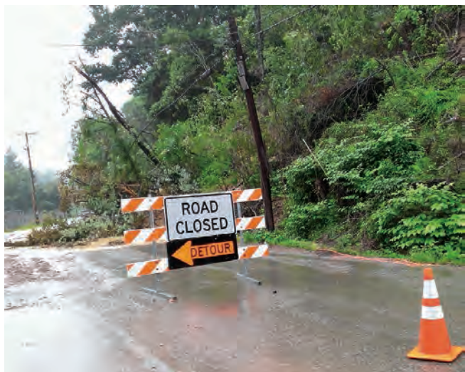
Abandoned Mine Landslide, Kentucky
