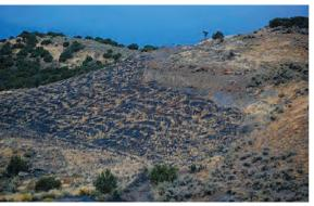
Construction at the fire occurred over an area of approximately 5 acres, and resulted in the excavation and quenching of approximately 168,000 cubic yards of material. The Skull Creek fire was completely excavated and cooled in approximately 7 months. Following replacement of the cooled material, the site was recontoured to natural slopes and revegetated.
